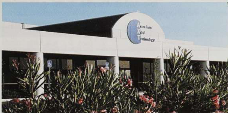
Figure 1. AXT's GaAs and InP manufacturing facility in Fremont, CA
