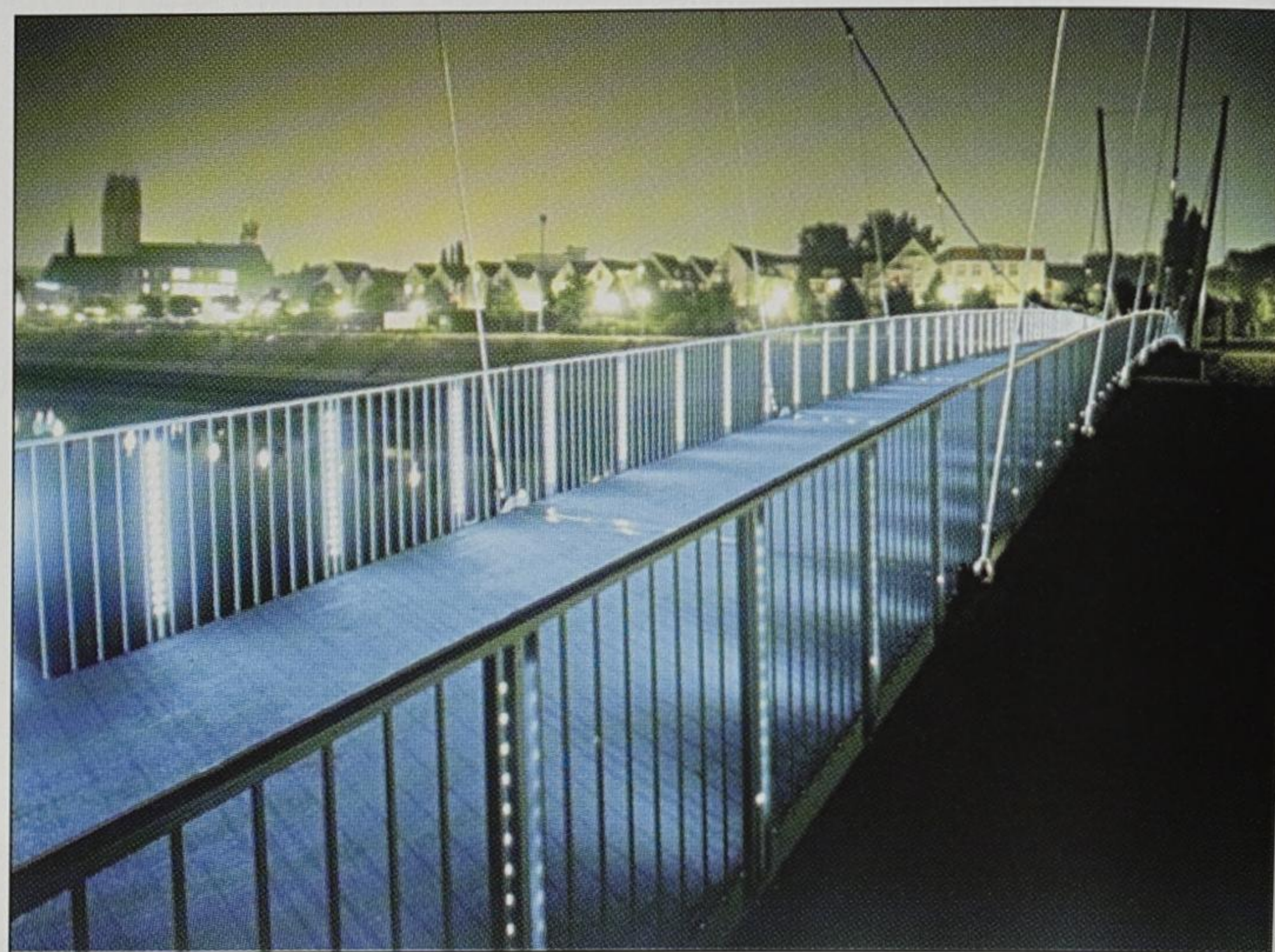
140 vertical strips of white LEDs illuminate this 70-meter-long bridge in Duisburg, Germany.
