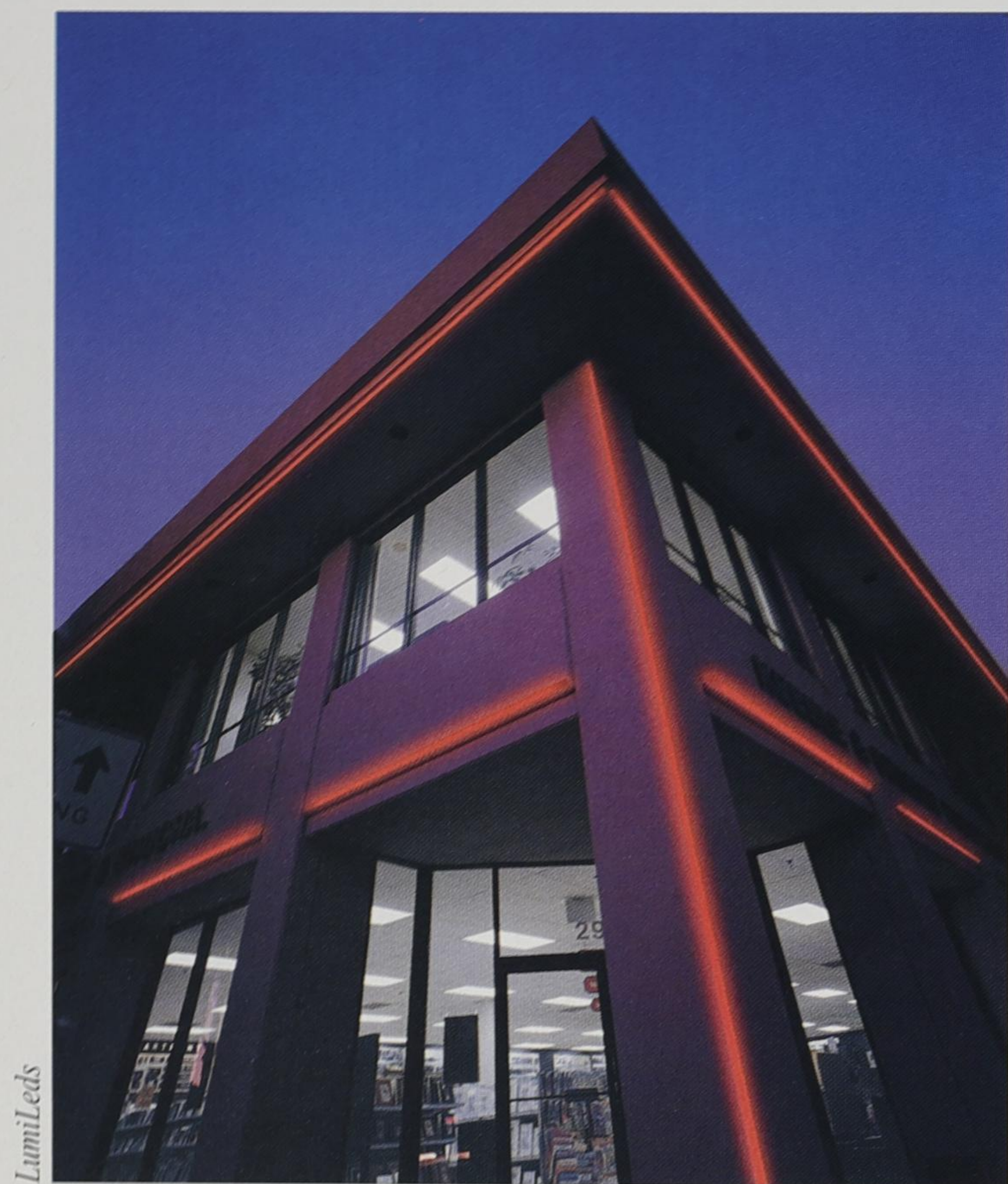
Figure 1. LumiLeds' chip-strip lighting can be used as decorative illumination on the edge of strip mall shops and buildings.
