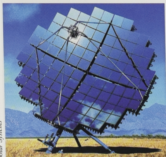
Figure 2. This 20 kW dish, installed in Fosterville, Australia, by Solar Systems is a prototype of the 24 kW systems that will soon be installed elsewhere in Australia. The receiver uses silicon concentrator cells made by SunPower and has an area that is 1/500 of the dish area.
