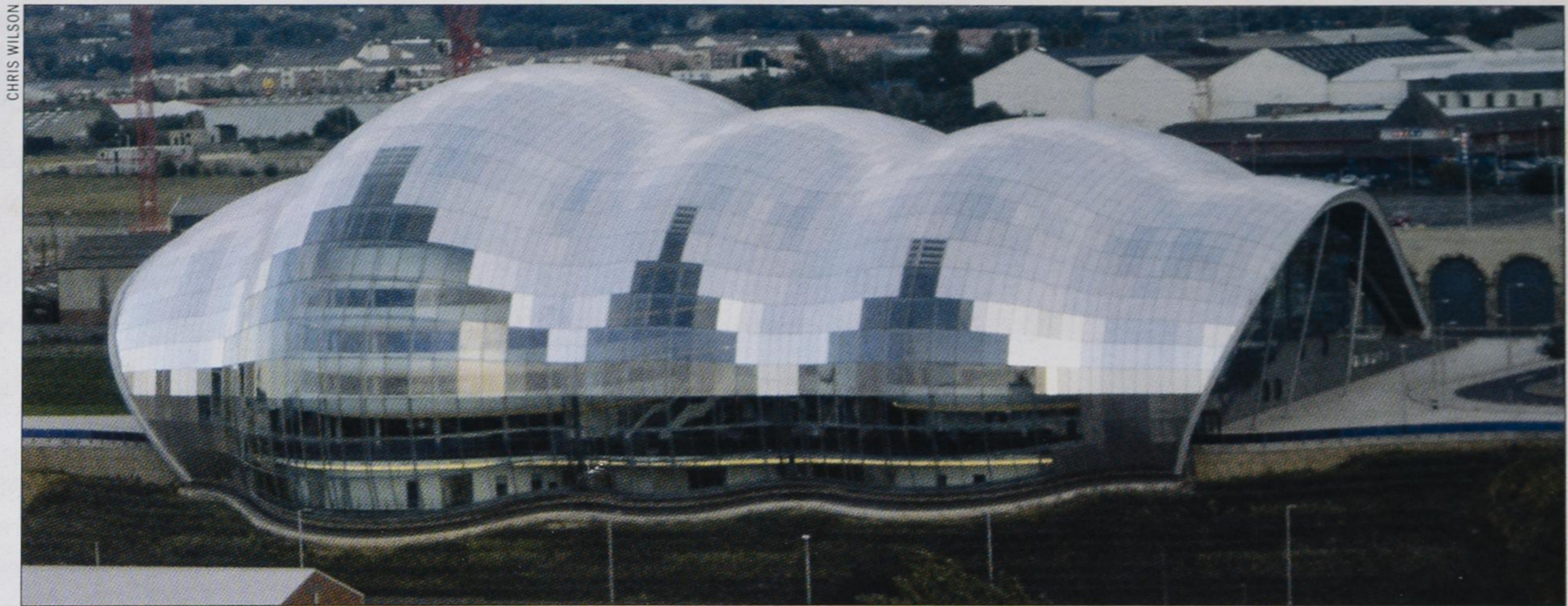
The Sage Gateshead , by the River Tyne in Gateshead, was the venue for this year's ECSCRM conference. The building opened in 2004.
