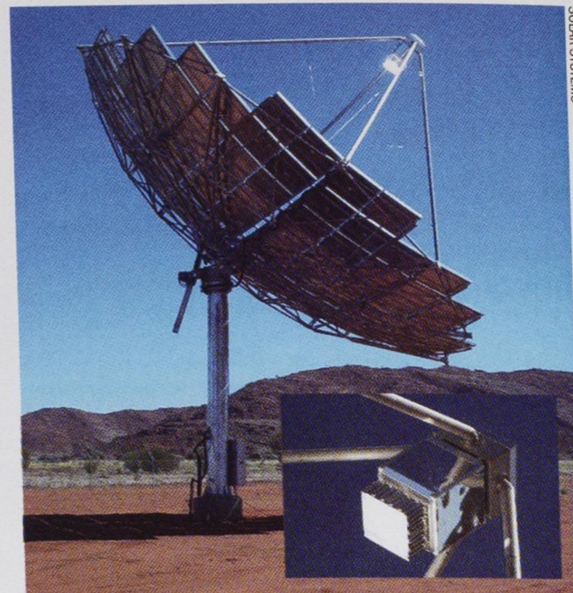
The concentrator dish at Hermannsburg featuring Spectrolab cells has been operating since April. Inset: the element that houses the triple-junction cells.
