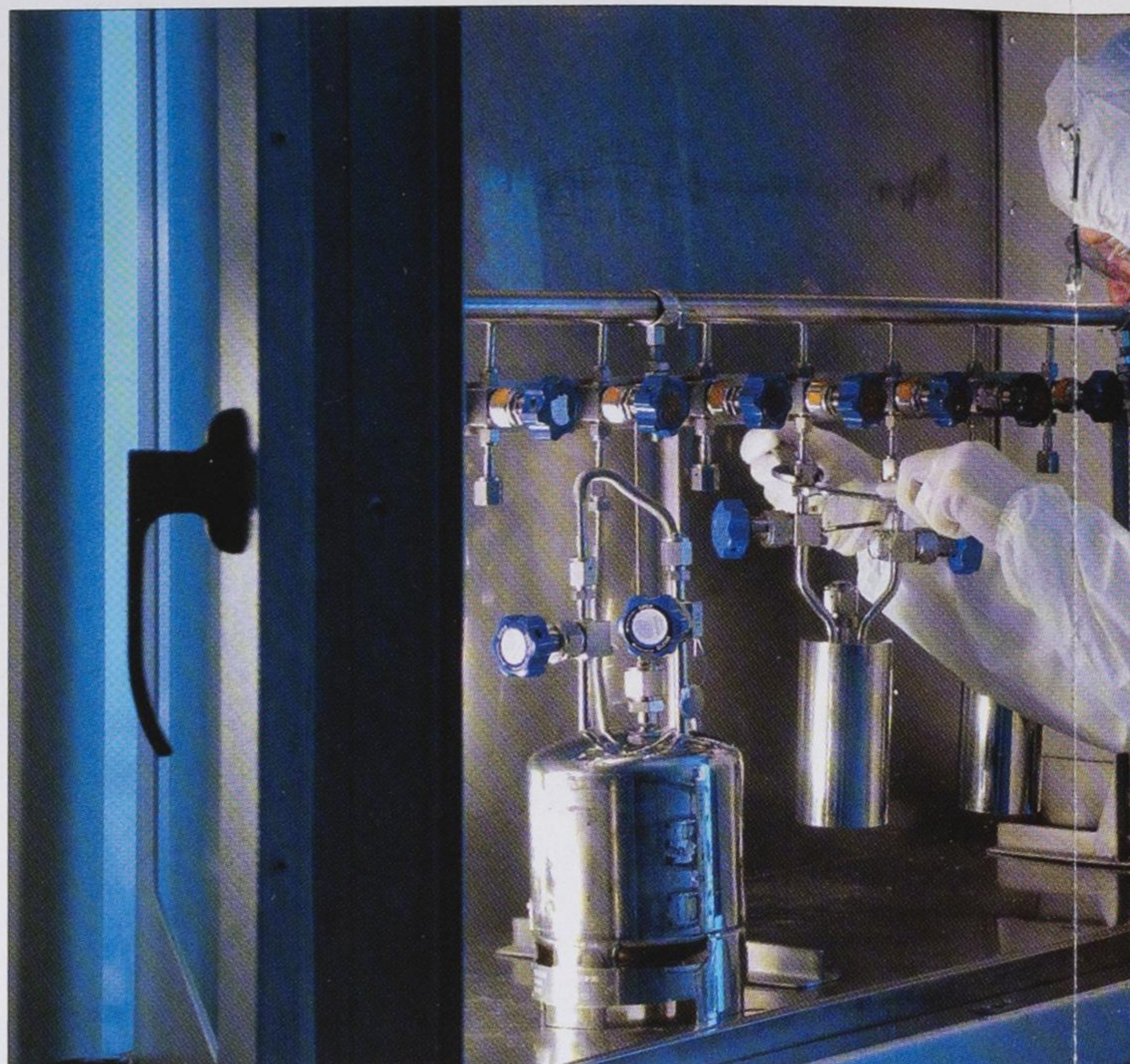
SAFC Hitech has around 1000 designs of bubblers on file (above), but it is now e systems. Although its trimethylgallium plant (right) has a current output of around t
