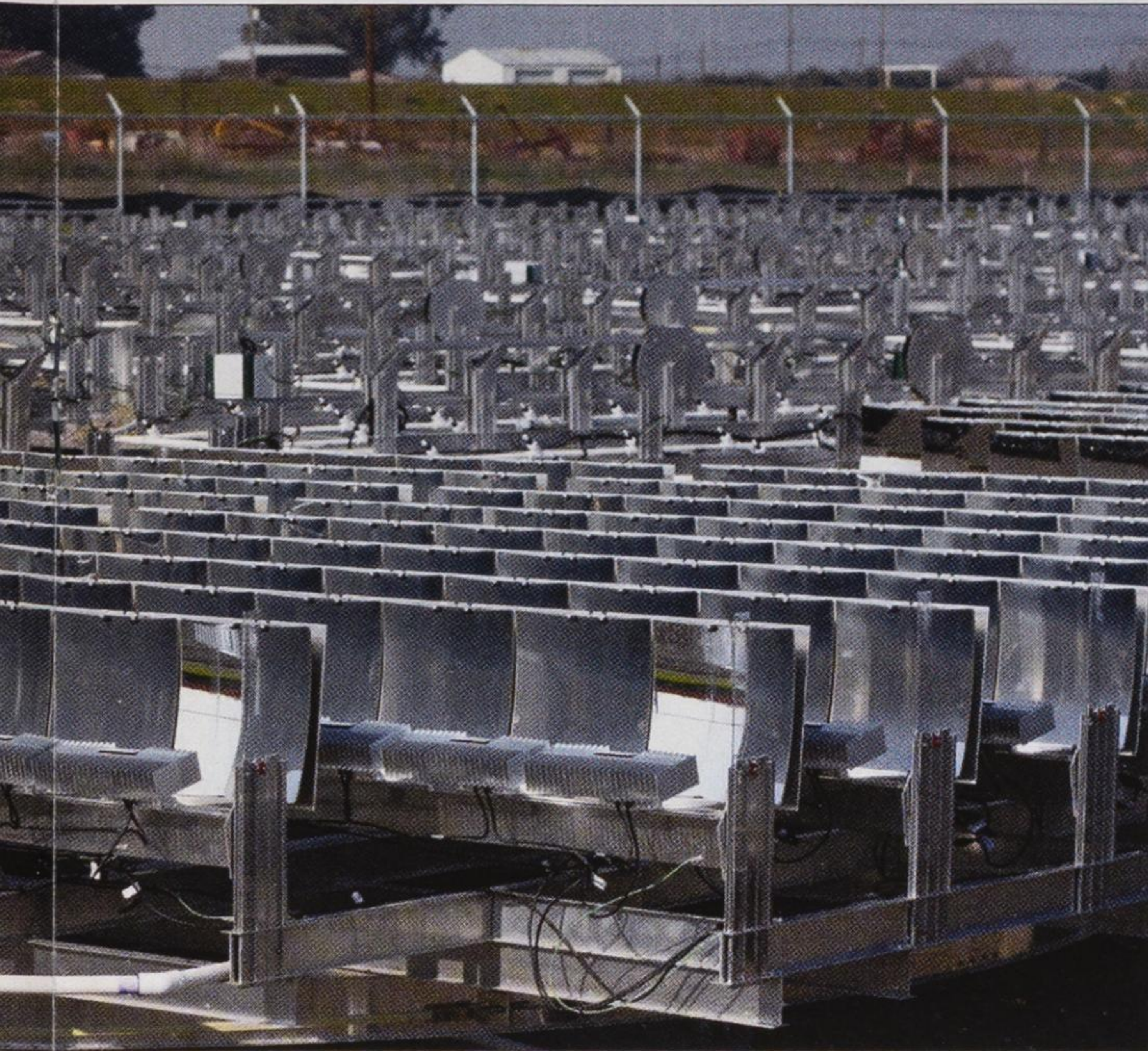
California. This large plant will feature hundreds of 3 kW, two-axis metal-framed parabolic mirrors to focus the sunlight onto multi-junction photovoltaic cells.
