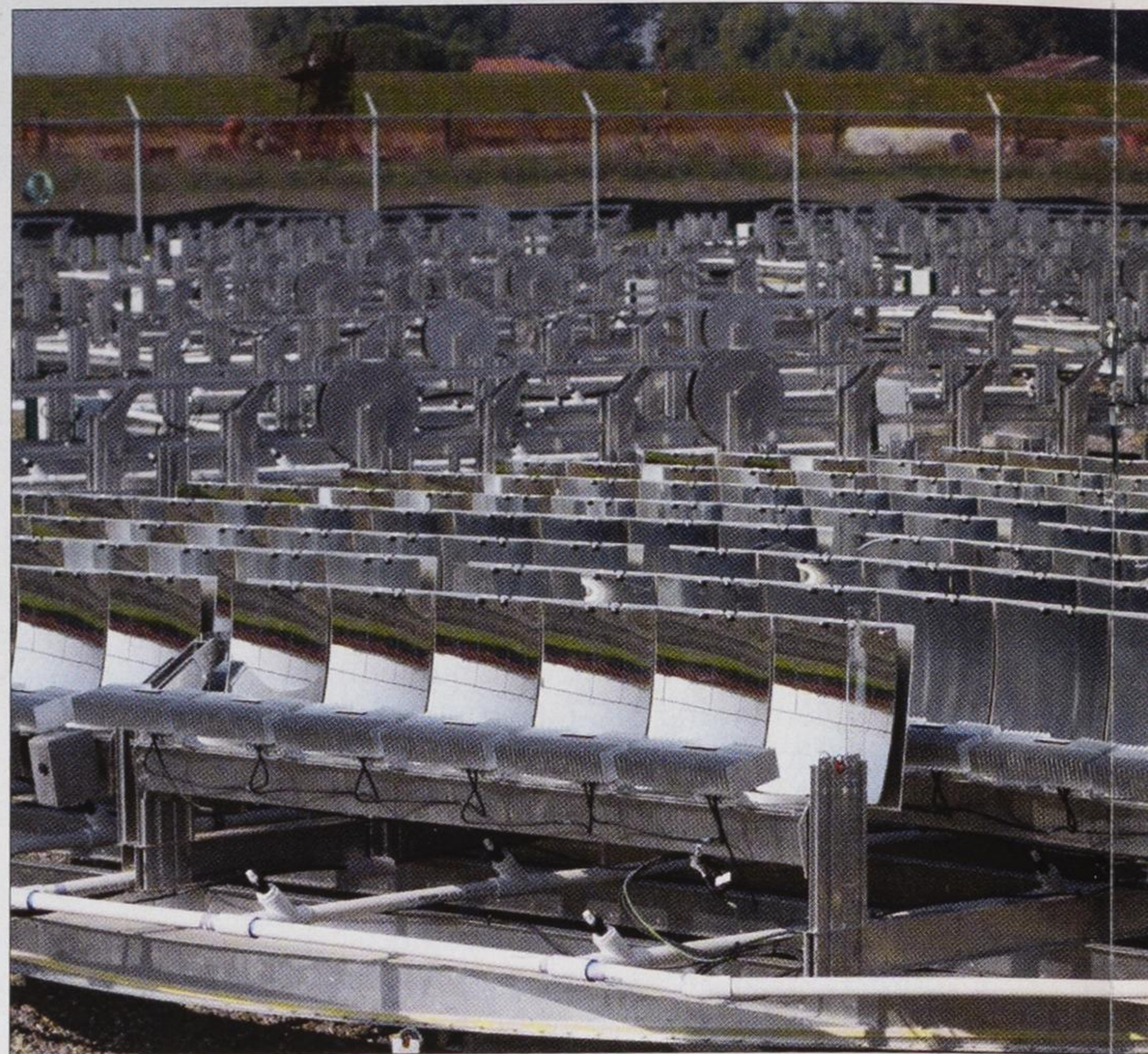
GreenVolts is constructing a 2 MW facility on an 8 acre site in Tracy, California trackers, with a diameter of nearly 6 m. Electricity is generated by using parabolic
