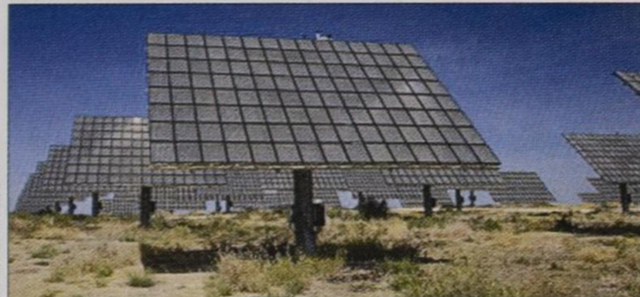
Concentrix Solar's installation at Casquemada, near Seville in Spain. Under clear skies, the plant operates at an AC efficiency of 23% – equivalent to the record conversion first achieved last year.
