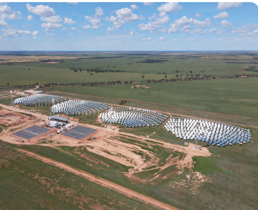
► Figure 4. Four RayGen solar towers during commissioning. RayGen's storage construction is nearing completion and will be operating commercially in early 2023.
