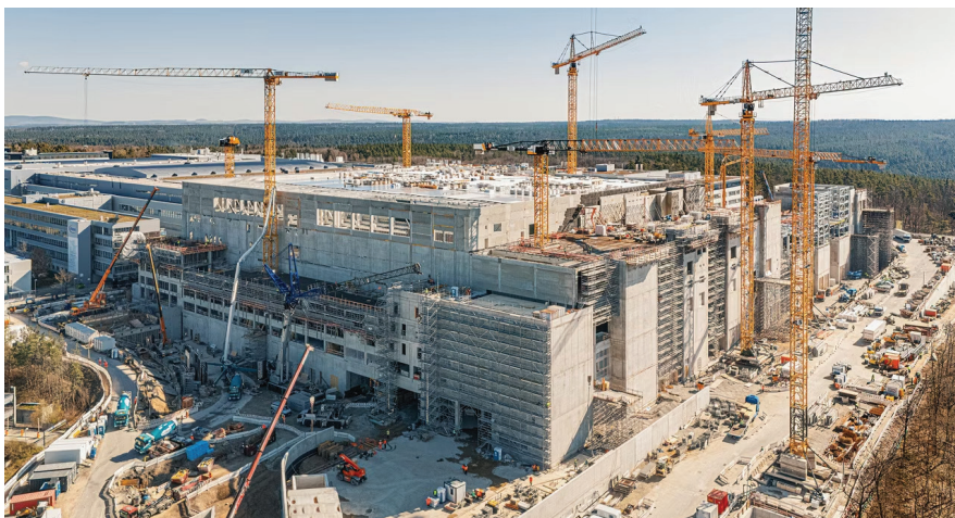
➤ Construction site of Infineon’s Smart Power Fab in Dresden. [Infineon]
