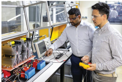
► Prasad Kandula and Marcio Magri Kimpara set up testing of ORNL-developed medium-voltage circuit breakers
