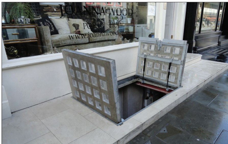
Pavement access flaps
