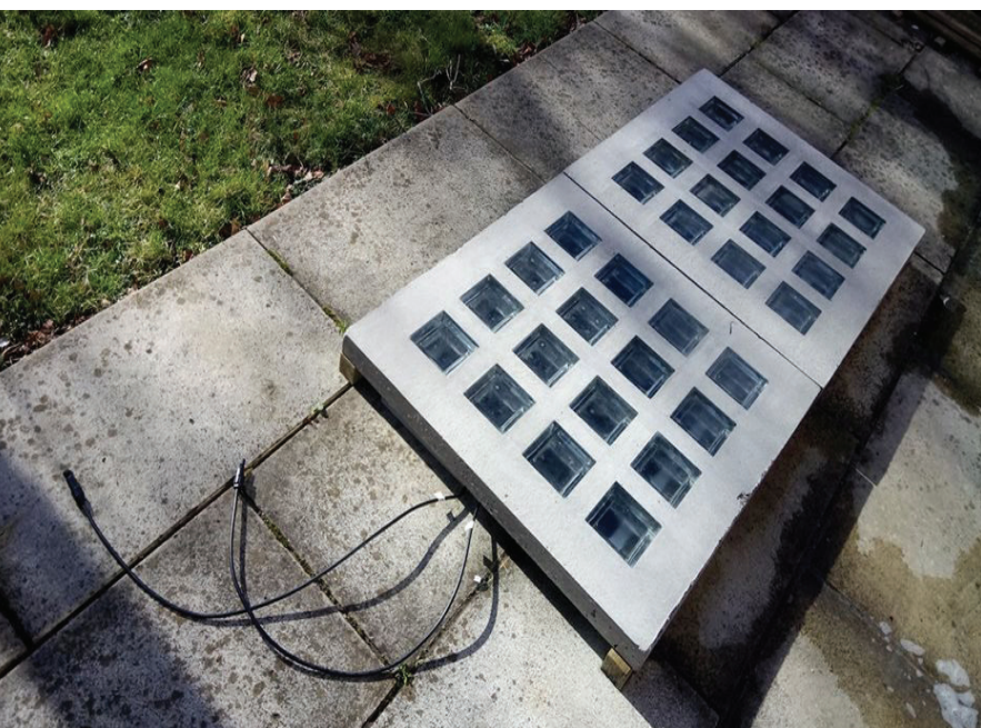
Solar sidewalk (C) test bed
