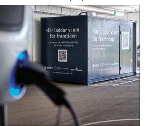
When an electric vehicle, after many years in traffic, is at the end of its life cycle, the battery still has a large part of its capacity left, sufficient for use in the energy storage systems built by BatteryLoop. So instead of sending the batteries for recycling, they get a second life.
