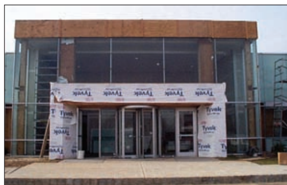
Anadigics' current headquarters under construction
