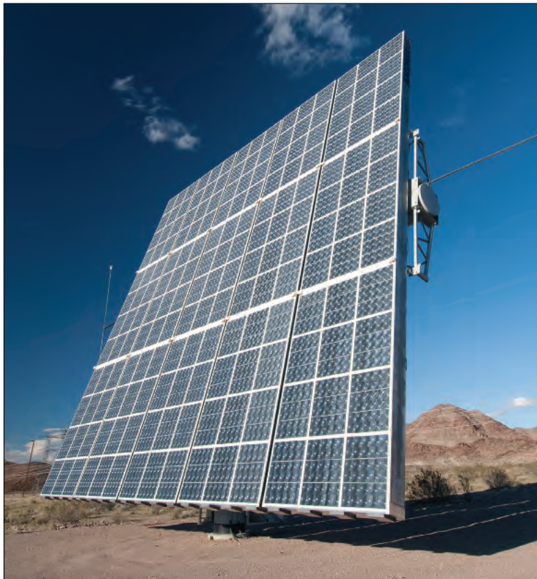
This summer Amonix completed its 240 kW CPV system deployment at the River Mountains Water Treatment Facility, Nevada. Recent efforts by this company also include a substantial expansion to its manufacturing capacity. Credit: Amonix.
