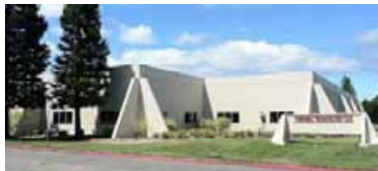
Thermal Technology's new production facility, which is dedicated to Model K1 sapphire crystal grower assembly
