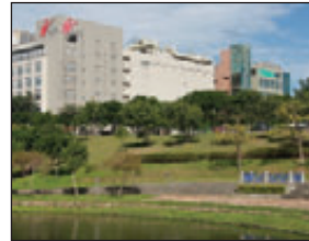
WIN's headquarters at Hwaya Technology Park on the outskirts of Taipei has two fabs with a combined capacity of 20,000 wafers per month
