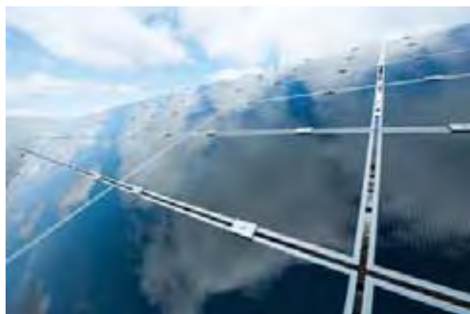
First Solar thin-film solar photovoltaic modules in a ground-mounted solar power plant
