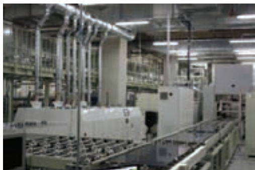
TSMC Solar S-Fab production line, located in Taichung, Taiwan
