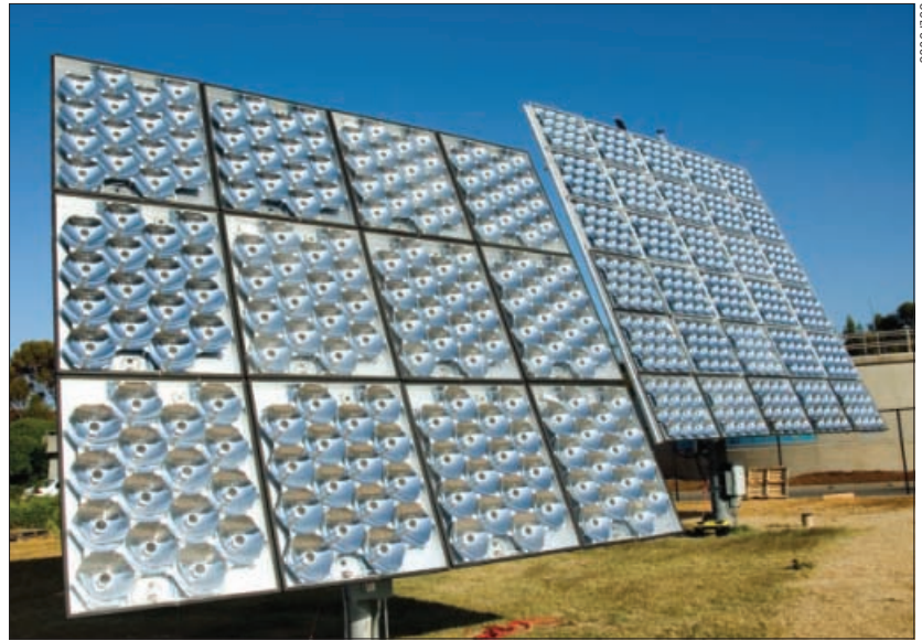
Quantasol's cells are designed for concentrator systems, such as those produced by SolFocus.
