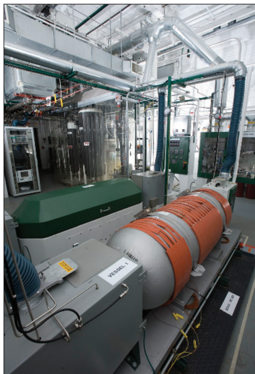
Figure 3: Ammonia Pilot Plant at Praxair's Technology Centre
