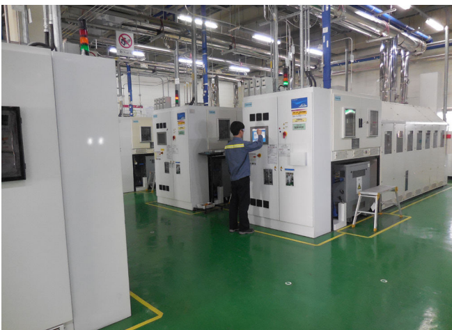
Generation-F ® zero global-warming potential, superlative cleaning efficiency on-site fluorine generators
