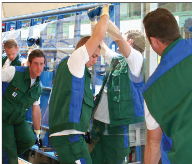
The trend towards triple insulation glazing and ever larger units is leading to high glass weights and placing greater requirements on the installation team. Photo: Messe Düsseldorf
