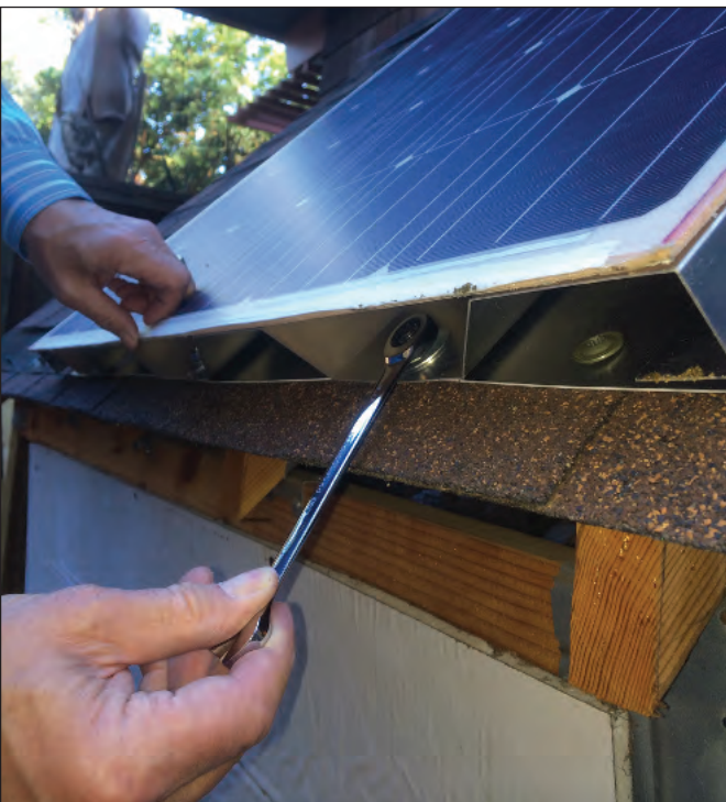
Figure 7 – Attachment of the module/support structure to the roof
